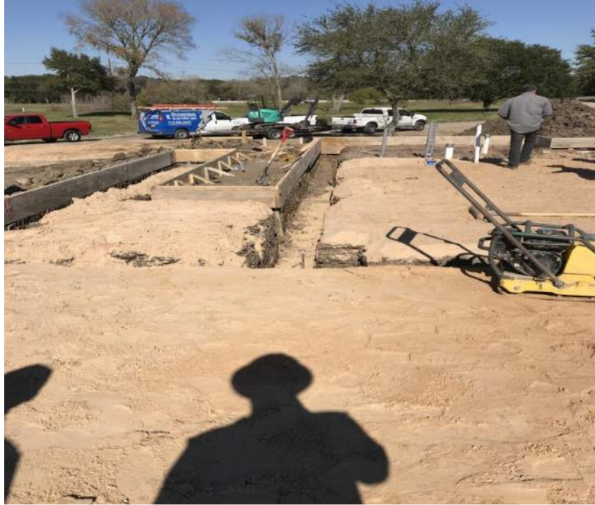
Grade beams for stage.
