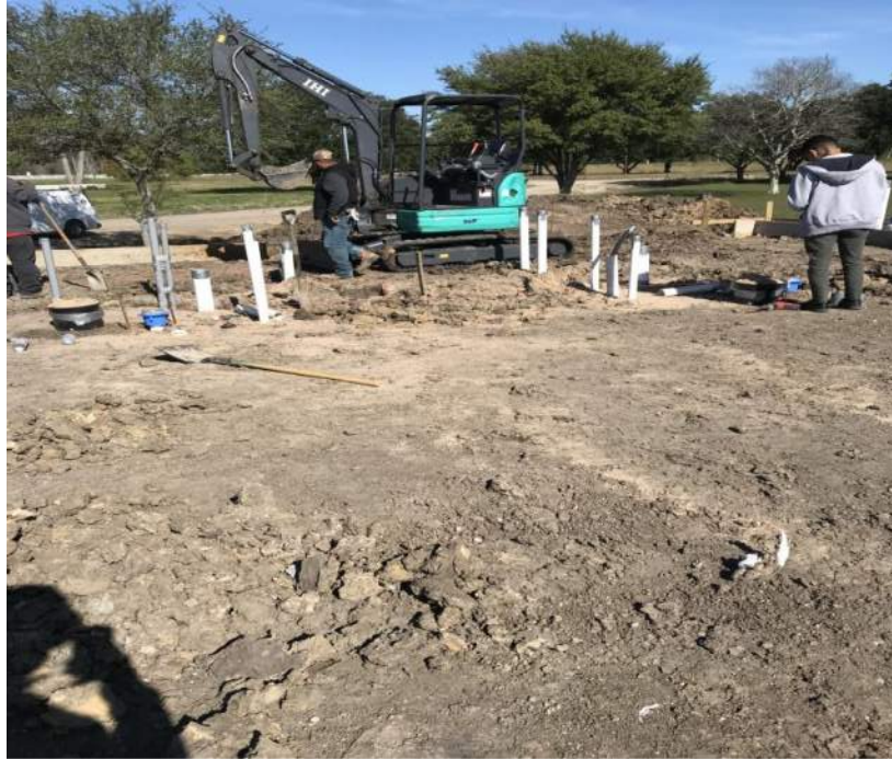
Stage Slab plumbing and electrical rough-in
