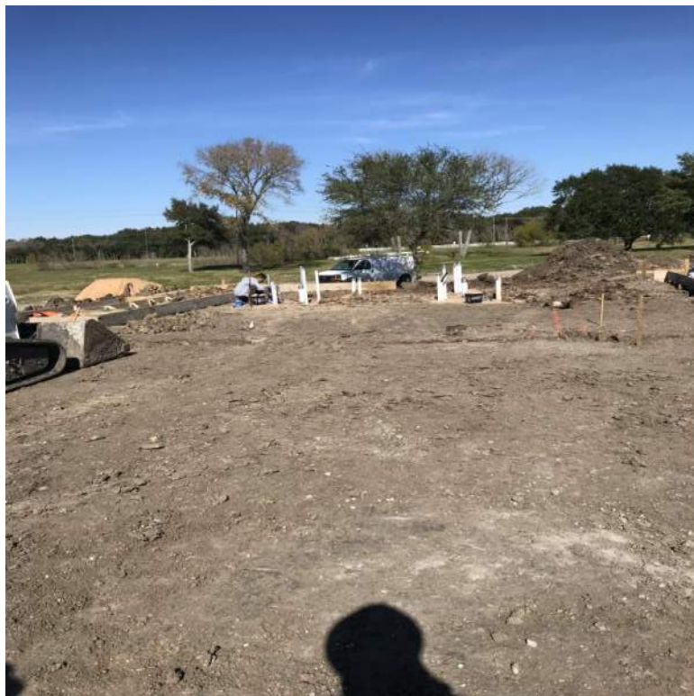
Grading for the stage slab
