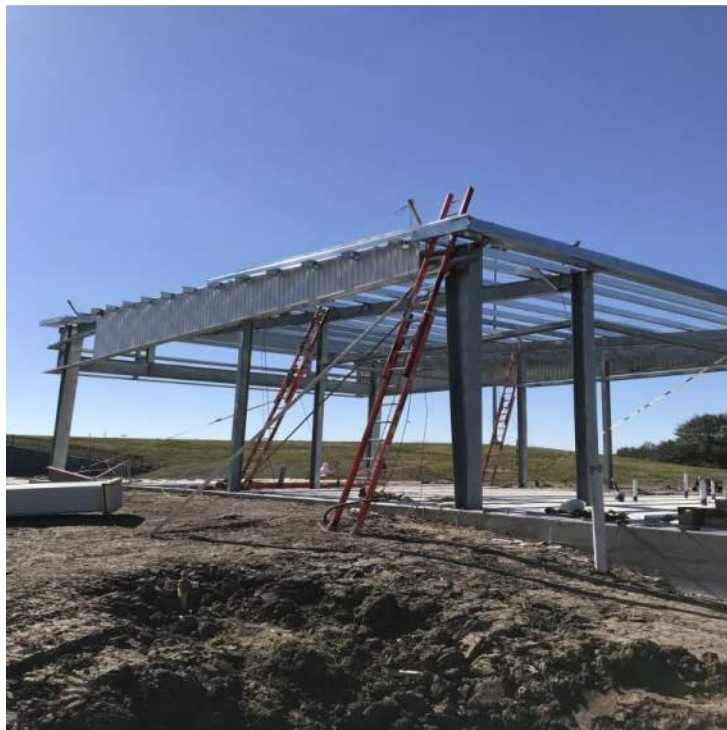
Erection of the stage
