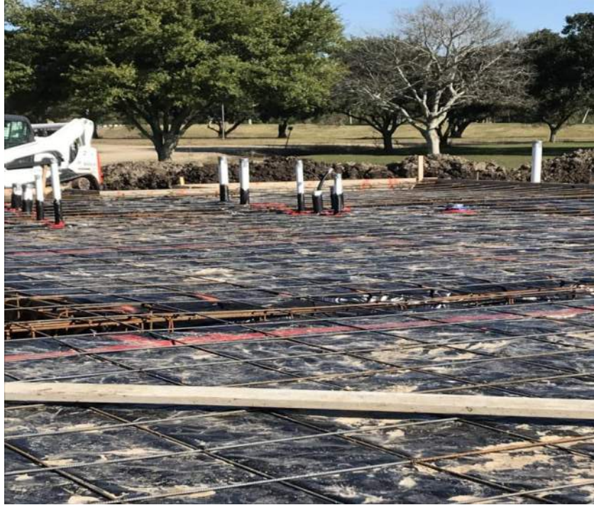
Vapor barrier and rebar installed
