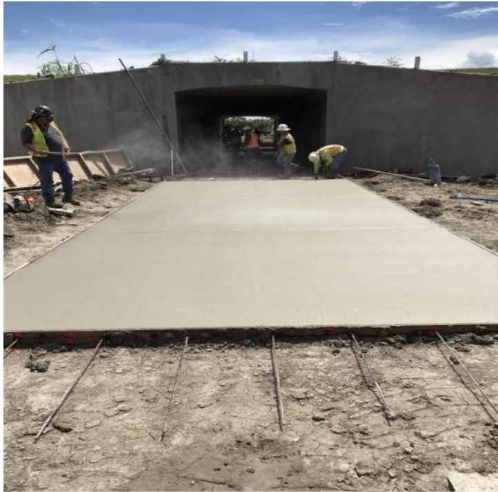
Concrete placement @ Tunnel
