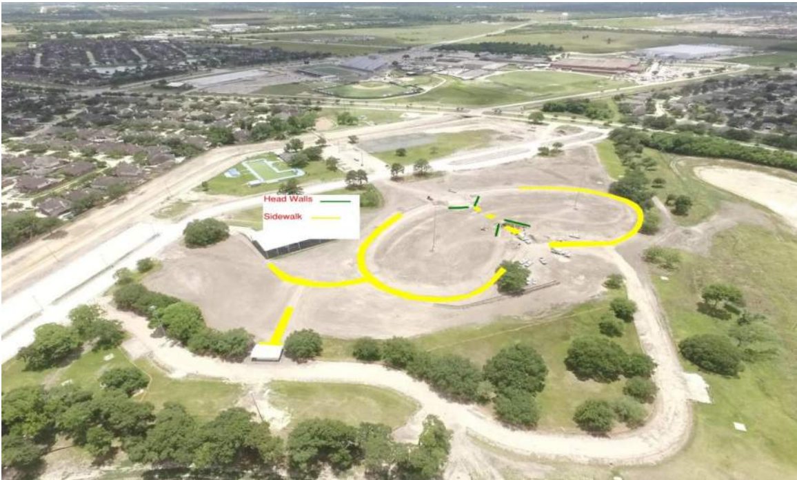
Areas of completed Concrete work
