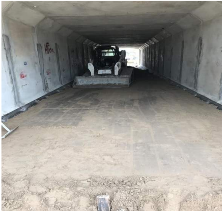
Stabilize sand used for grading inside the tunnel for sidewalk
