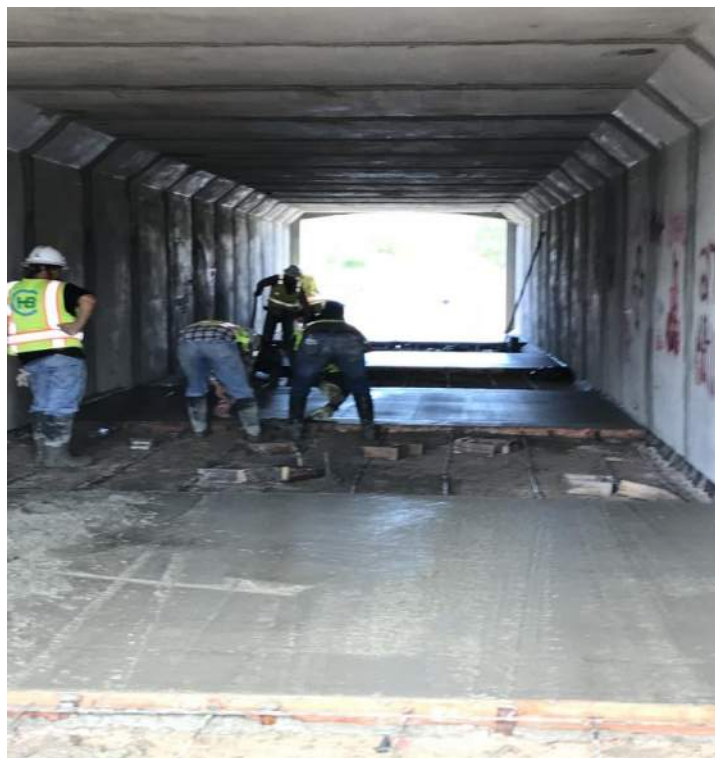
Concrete placement inside tunnel
