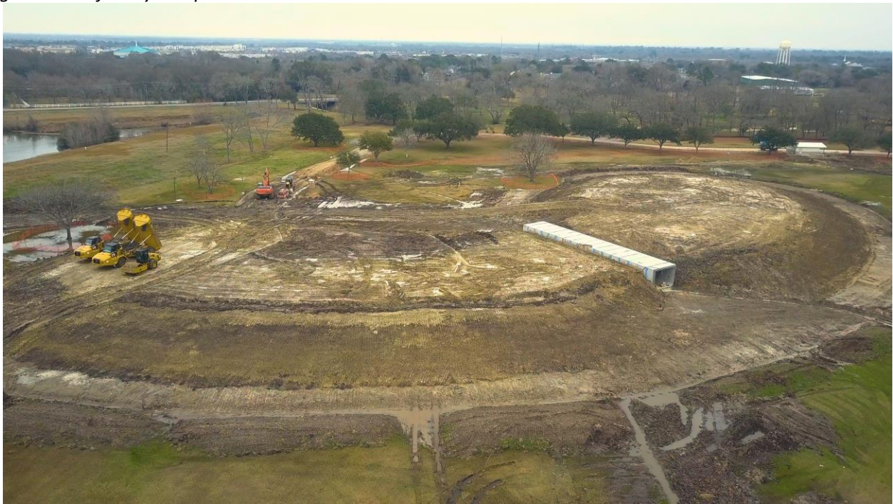
Build-up of earthen berm amphitheater
