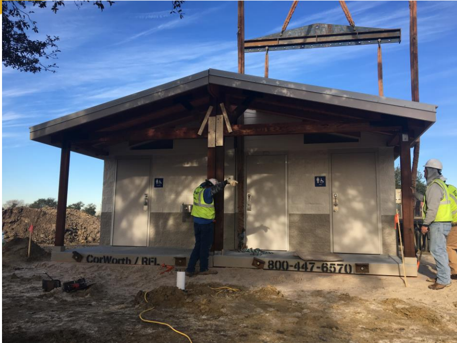
Joining restroom facility components
