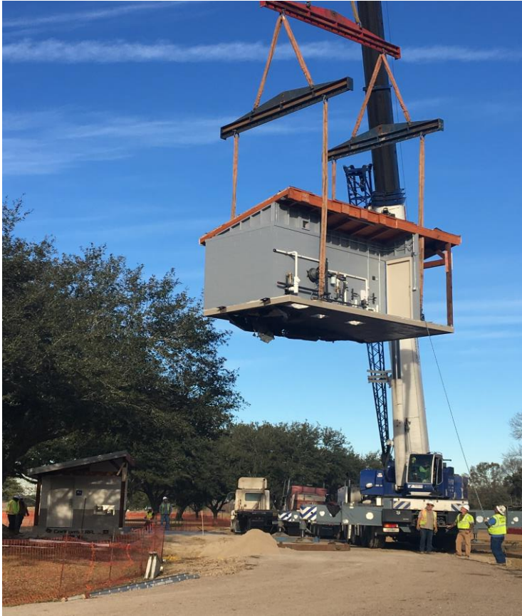
Installation of restroom facility using a crane to place components
