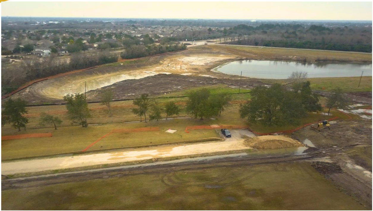
Expansion of detention pond
