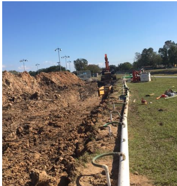
Pumping groundwater in preparation for installing new sewage line
