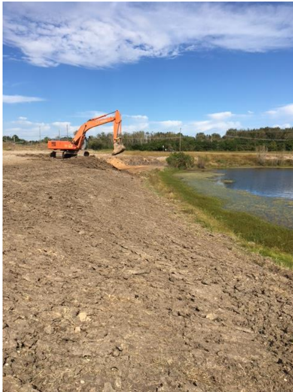
Beginning excavation of pond.
