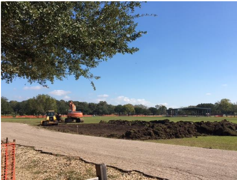
Beginning earthwork to build berm
