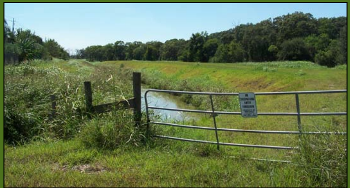
Access gate to Drainage District maintenance easement
