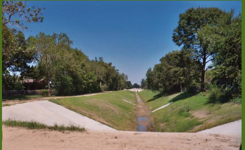
A north-south drainage channel through the Corrigan South neighborhood could accommodate part of a trail segment linking Corrigan Park to the north and Centennial Park to the south and east.
